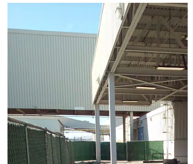
Above left and below are examples of vehicle conveyance trestle
